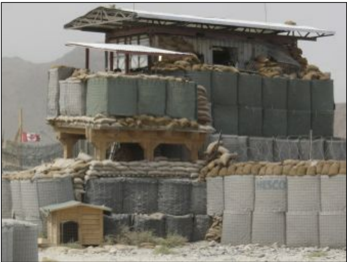
BELU ISAF 6-01, bunker met observatiepost op Kabul International Airport
